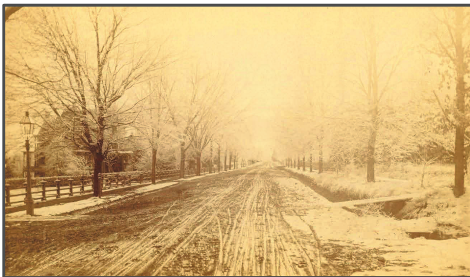
Figure 11: View Along South Mountain Avenue from Myrtle. Note the excavations on the right for sewer/water installations. (Montclair History Online—Digital Photo Collection # P2568).
