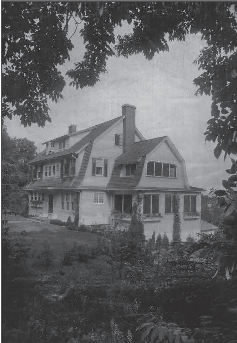
Figure 29: Dudley Van Antwerp designed Dutch Colonial Revival dwelling on Lloyd Road exhibiting English Arts and Crafts influences (e.g. shed dormers, corbeled chimney caps, etc...). (Montclair History Online—Digital Photo Collection # P2517).
