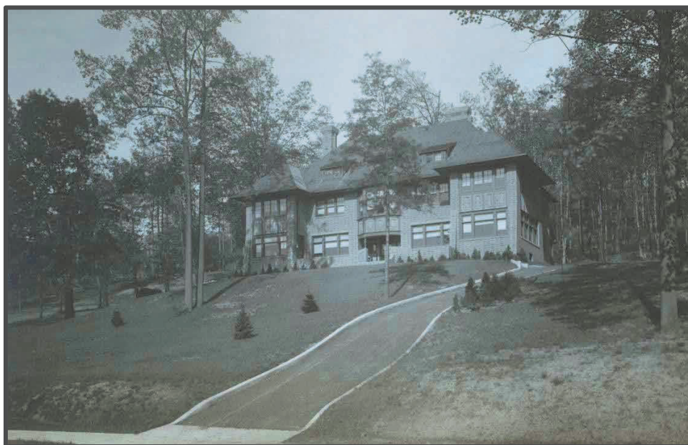
Figure 27: Residence at 70 Undercliff Road exhibiting Arts and Crafts influence (high hipped roof, shed dormers, decorative chimney caps, oriole front entry, etc...). (Montclair History Online—Digital Photo Collection # P2722).
